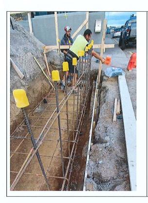
Excavation to base of footing depicts firm good-ground in accordance with foundation requirements.
