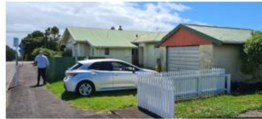
View of existing garage from street outside neighbouring site, 107 Morley Street.
