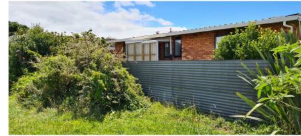
Eastern boundary to 47B Barrett St, corner of section
