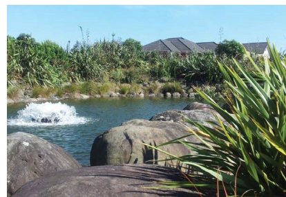
Example of stormwater detention pond designed as a landscape feature integrated into the subdivision's open space.
