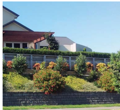
Retaining walls split into levels and planted integrates well with the streetscape.
