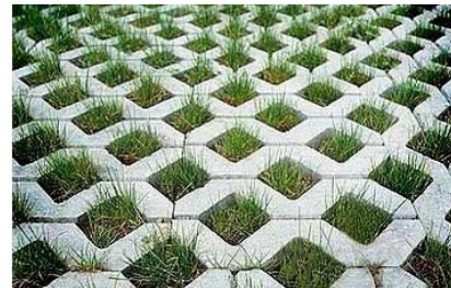
Use of permeable paving reduces visual impact of driveways.
