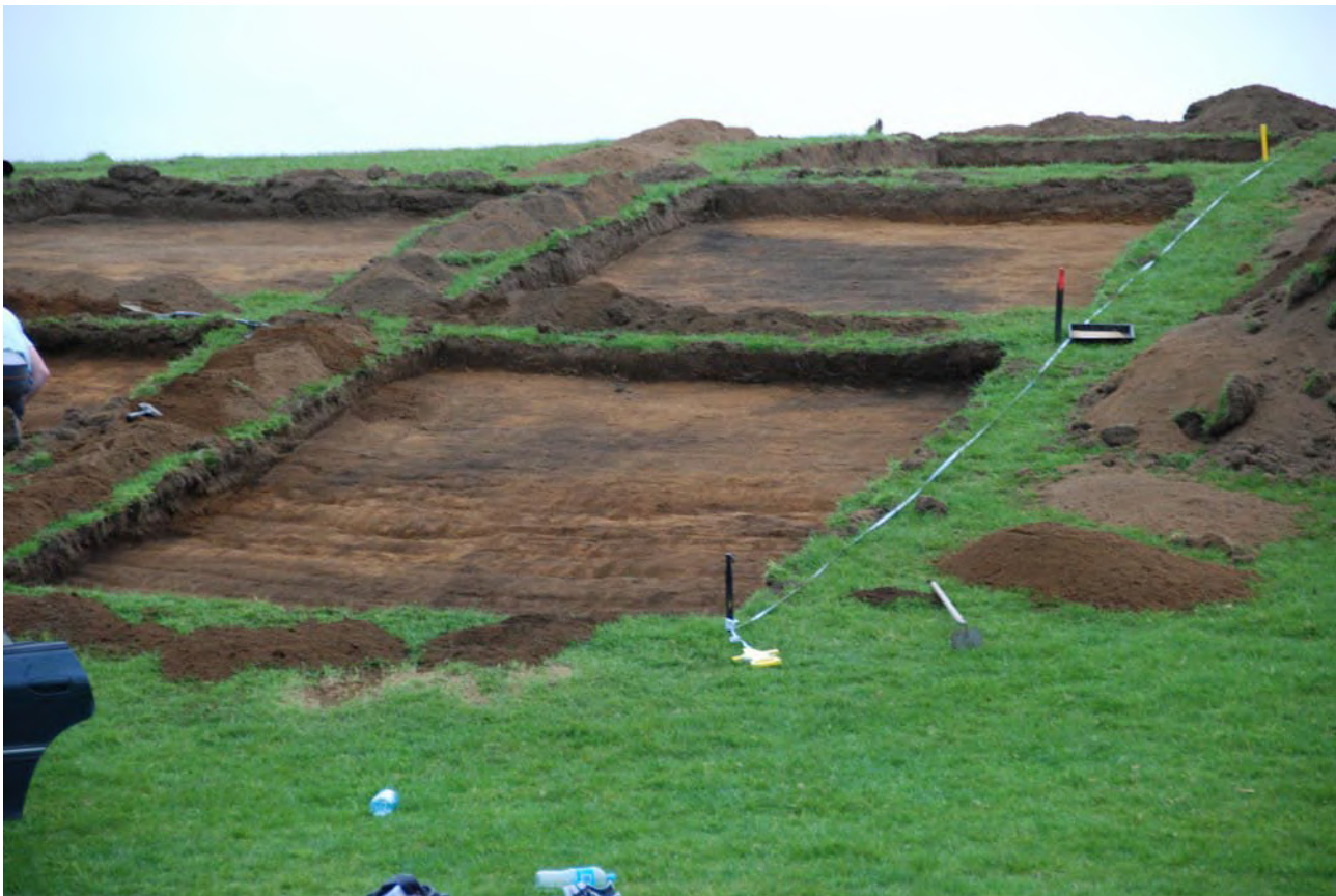
Fig.5: Initial topsoil stripping showing burn-off areas.
