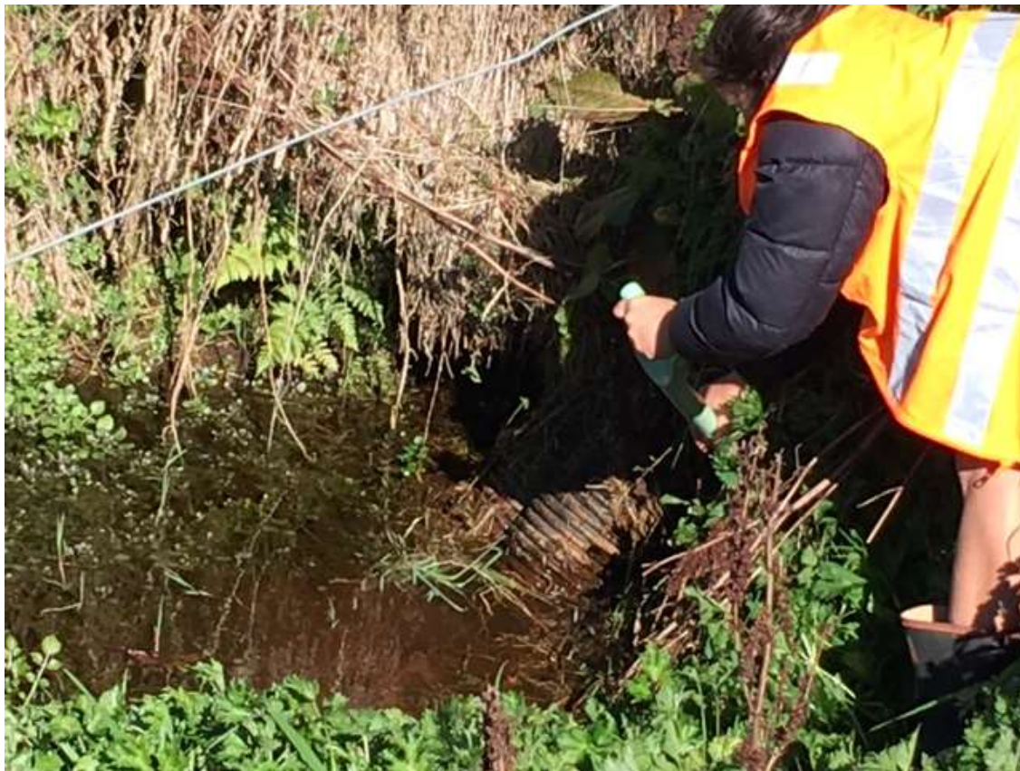
Figure 4: Drainage coil discharging to waterway
