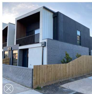
Lack of articulation and windows only addresses one street, creating a blank interface on secondary street.
