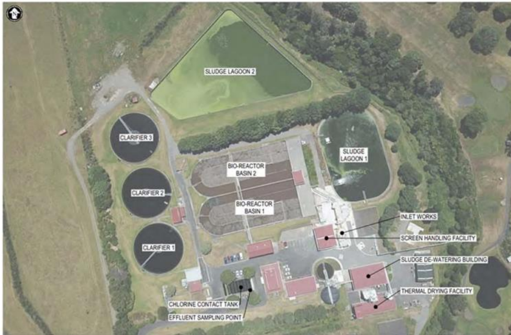
Figure 9 - New Plymouth WWTP Processes
