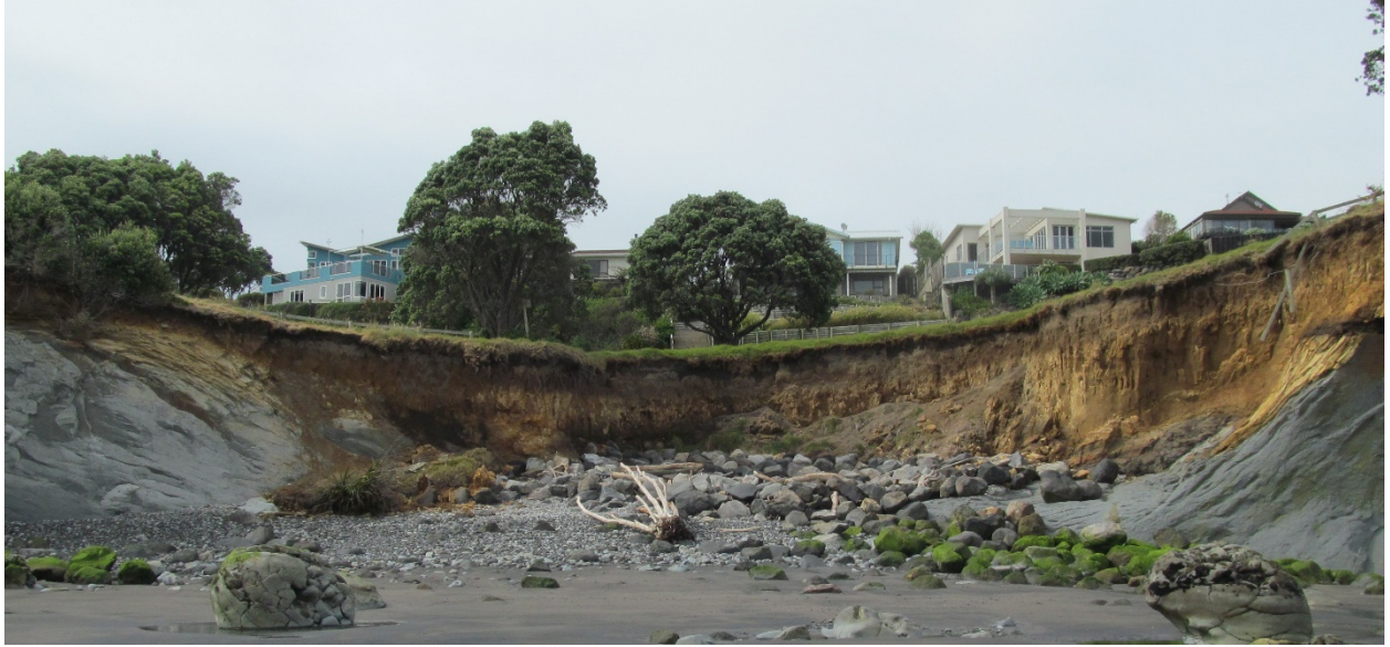
Coastal Erosion at Motukari Reserve, Onaero
