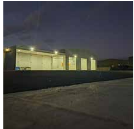
Construction of New Plymouth Transfer Station on Colson Road.
