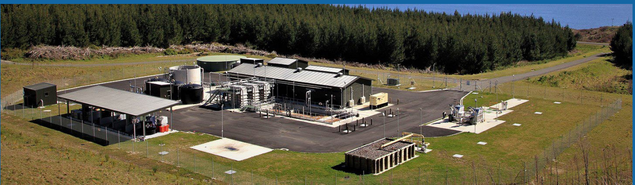
Rotoiti Rotomā Wastewater Treatment Plant
