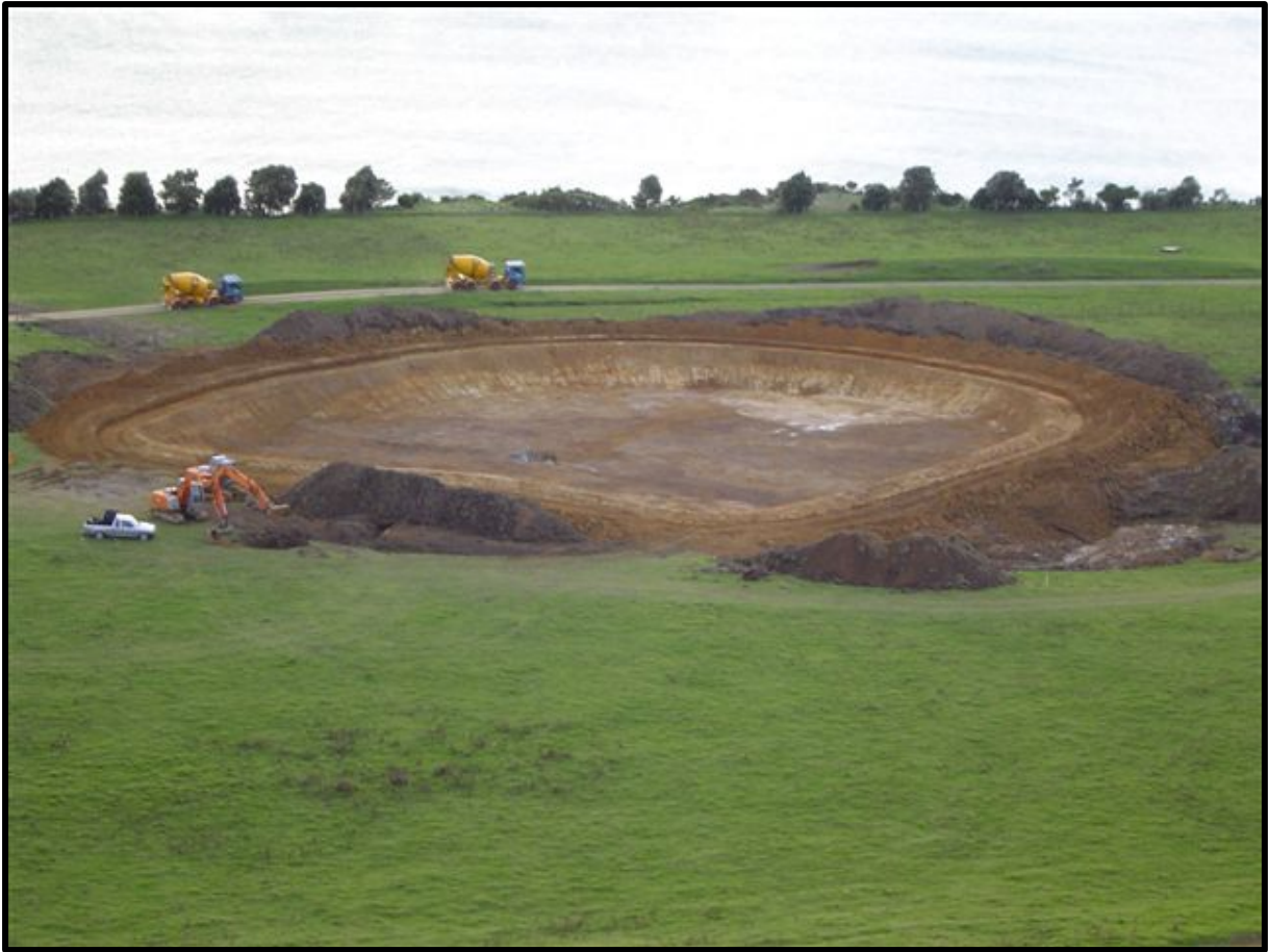
Pirikau pipeline relocation project May 2006. Excavation for water reservoir.
