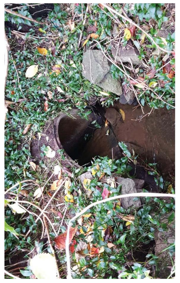
Photo 1. Inlet end of the existing 600mm diameter culvert pipe for the Wairau Stream Tributary flowing under SH45. Low flow situation.
