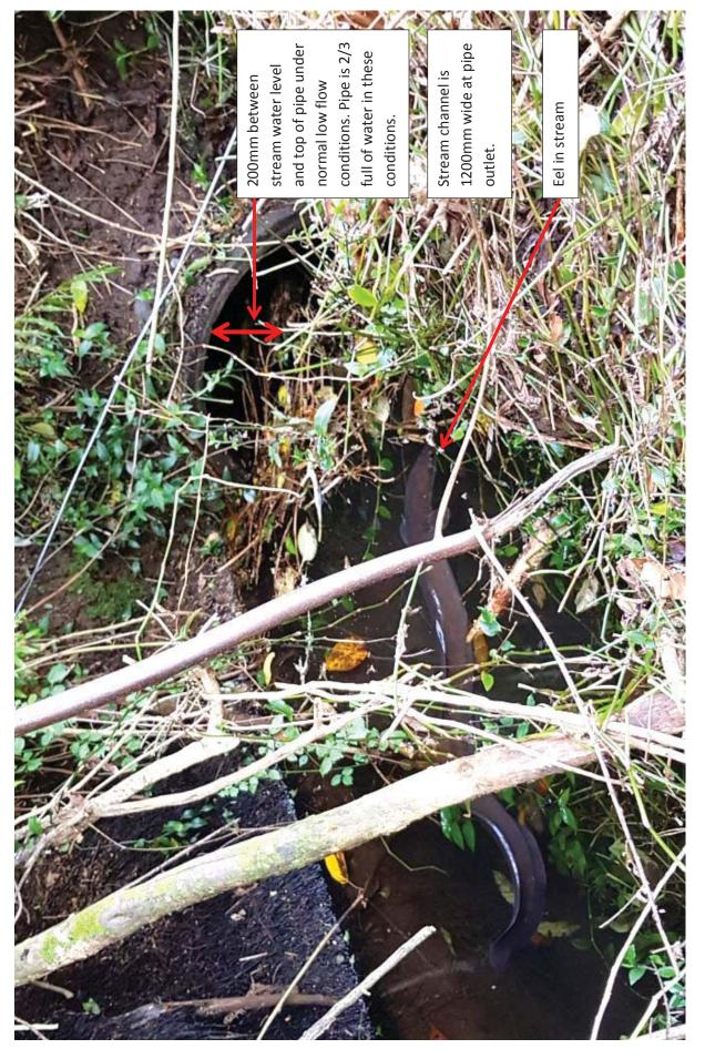
Photo 1. Outlet end of the existing 600mm diameter culvert pipe for the Wairau Stream Tributary flowing under SH45. Low flow situation.
