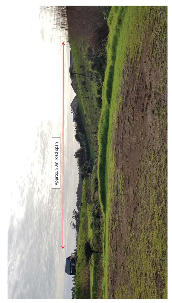
Photo 4. Wairau Stream Tributary gully at the point where the road into the proposed WES subdivision will cross. The new road will be 20 meters wide, maximum slope of 10% and will span approximately 80 meters between east and west banks.
