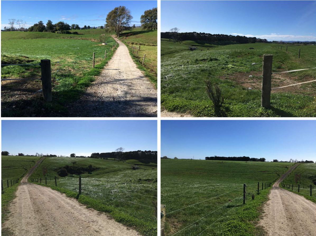
Figure 8: Track and gateway condition.
