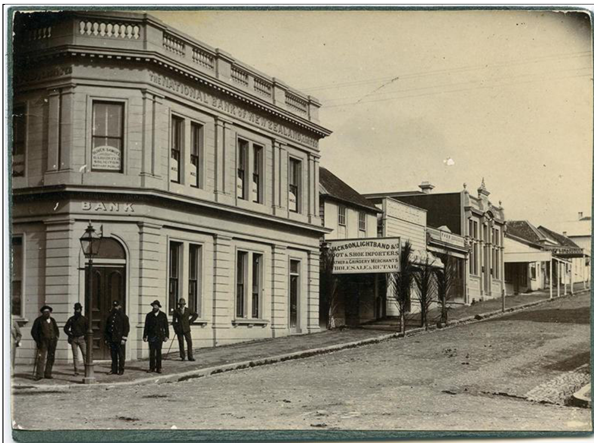
Figure 9: Brougham Street looking south with buildings on Town Section 683 at rear prior to 1885 fire. Unknown Photographer. "Brougham Street from Devon Street Corner". Circa December 1884. Puke Ariki.
