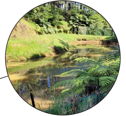
Silt control pond
