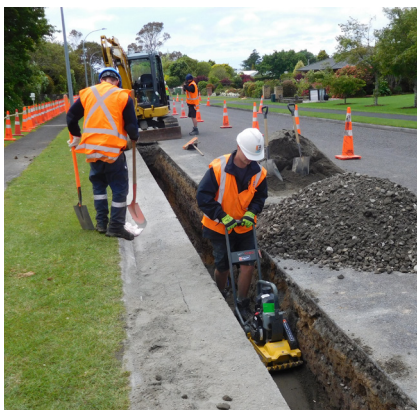
Inglewood's water runs clear again as a $10m project to replace the town's water pipes over three years is completed.
