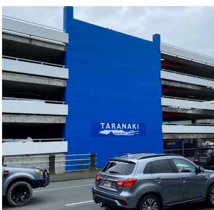
We allocated over $5m to earthquake strengthening the Downtown Carpark building so it can be re-opened for public use.
