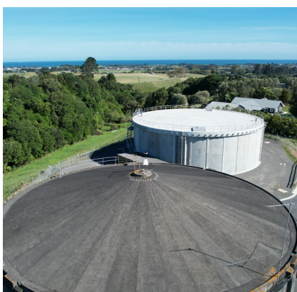
Two drinking water reservoirs, costing $18m, completed at Henwood and Mountain roads to supply Bell Block, Waitara, Lepperton and further north.
