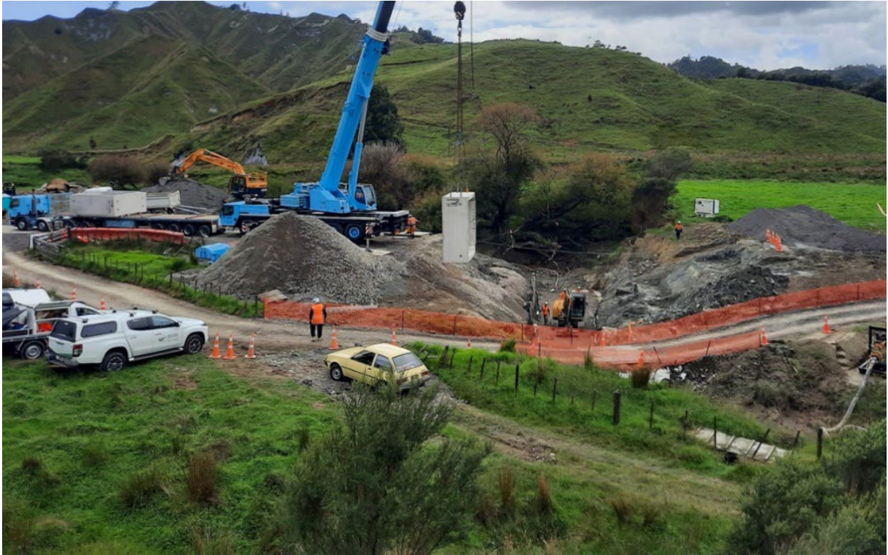
Figure 1 - Okoki Road Culvert
