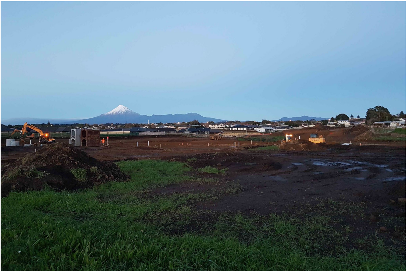
Parklands Road to Wills Road extension development
